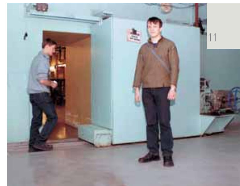
The entrance to the accelerator room is barred by an enormous one-meter thick lead door, an electric motor with a dashboard next to it. First, it is difficult to believe that something can move this metal “crag”. Then you insert the key, and there it is: the slowly moving door lifts the veil of the “accelerating mystery”.
